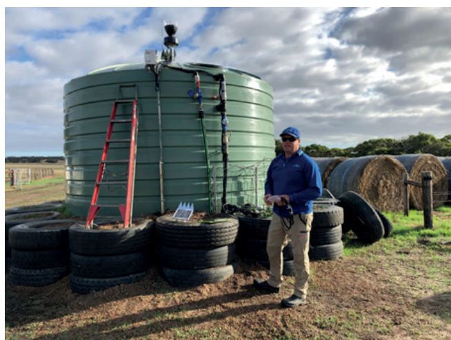
Figure 1: Shane (Alpha Group Consulting) and the tank monitoring set up. Note the gravel in the tyres to protect the tank and equipment from cattle.
